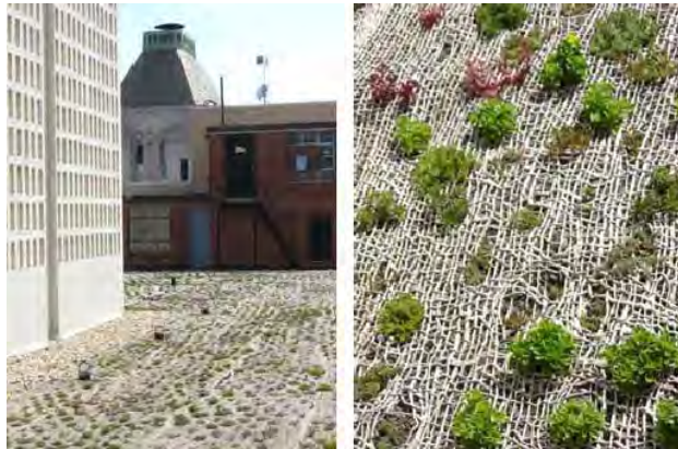
Figure B-2.8 Beginnings of a Green Roof
