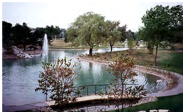
Figure B-2.7 Example of a Retention Basin Functioning as a Design Element
