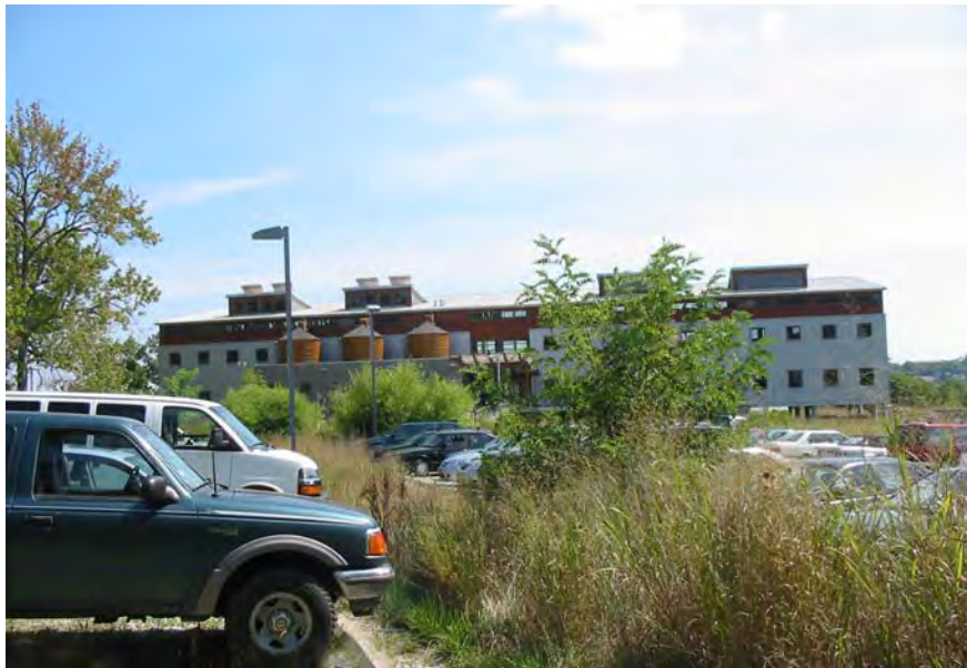
Figure B-3.5 Example of Parking Lot with a Permeable Parking Surface and Bioswales
