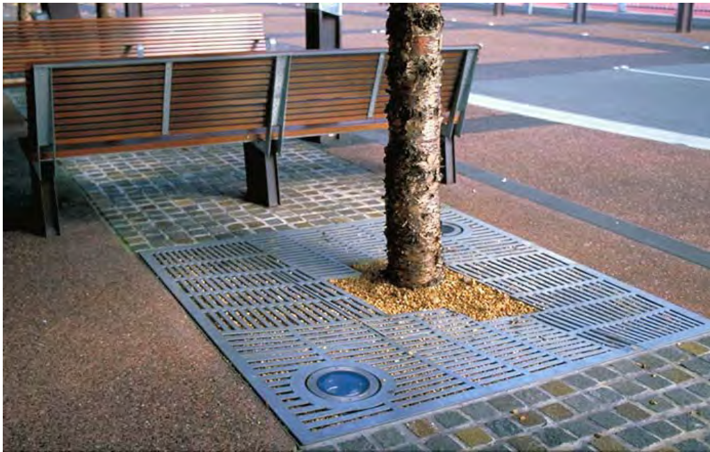
Figure B-8.3 Example of Tree Grate
